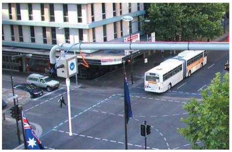
Mesh networking uses wireless nodes, like this one hanging from a pole, to provide wireless LAN coverage and wireless backhaul. The nodes interconnect to form a self-healing network or mesh that can support mobile data access, voice, cameras down a street, around a campus or over a whole city or community.
